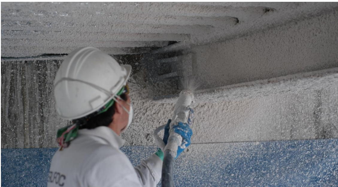
Picture 10 (Mortar spraying detail)
