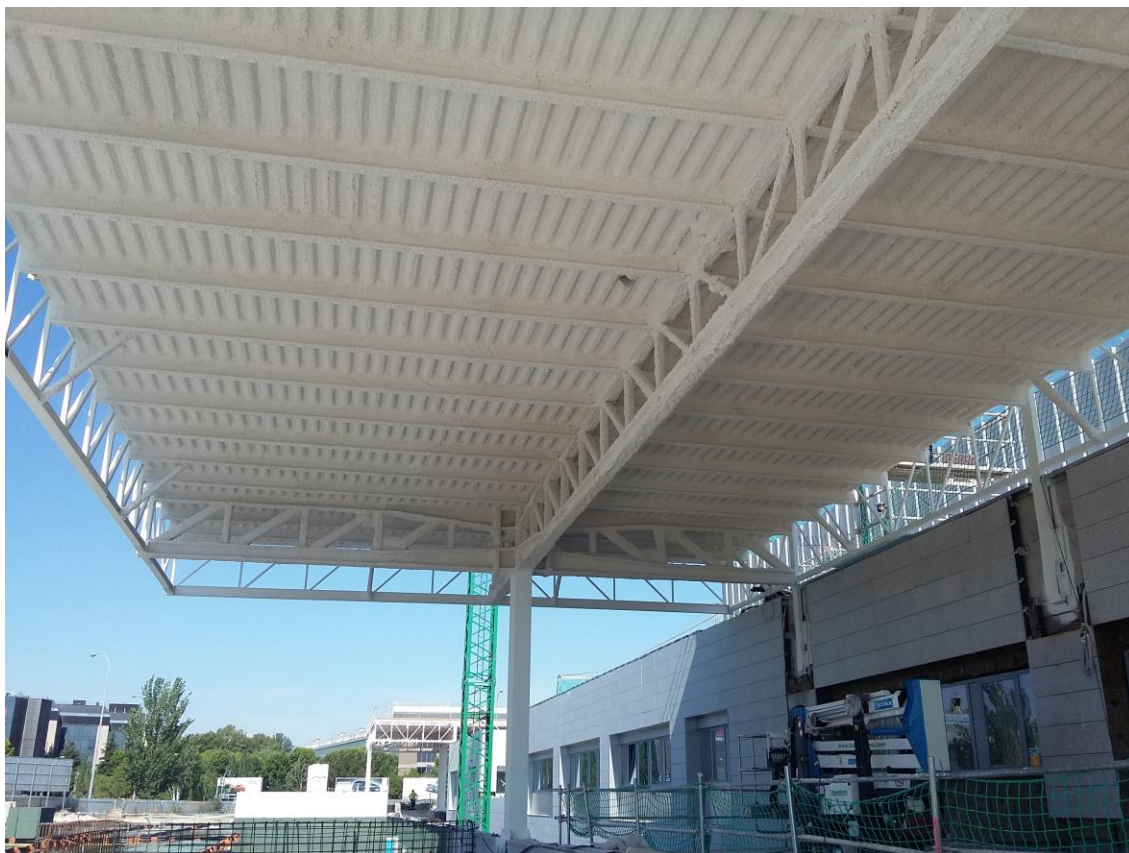
Picture 1 (Sprayed mortar on industrial warehouse)
